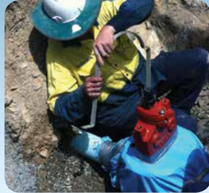
An InsertValve installation under full line pressure.
