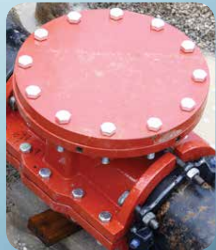
Blind flange installed.
