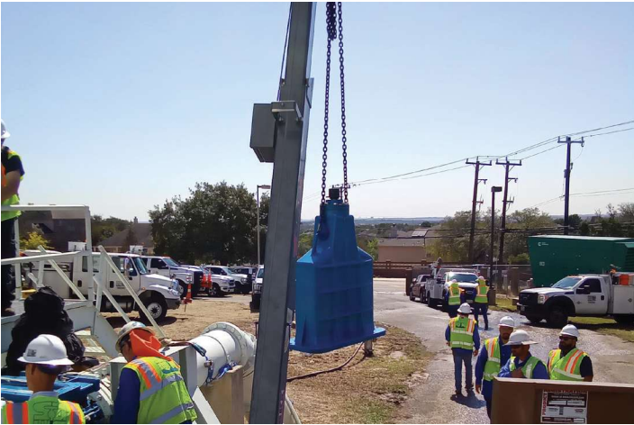
The bonnet was lifted into the valve body and secured in place.
